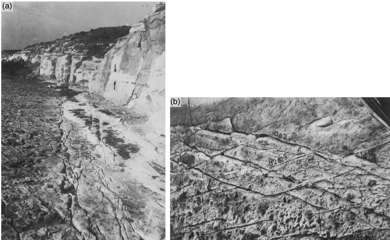
Fig. 6. (a) Chalk stratification and jointing in Middle Eocene chalks at Wadi Naim. Anastomose fractures of set 062^\circ (at centre of picture) cut through layers 1 and 2, and continue into the cliff. Note the irregularity in the floor and straightness of these fractures in the cliff. Arrows mark the thickness of layer 5 (60 cm) at the cliff. (b) Interaction between joints of sets 028^\circ (sub-parallel to the 30 cm scale at left-centre) and 062^\circ in chalk of the Horsha Formation (outcrop Y). Joints of both sets arrest at each other (at arrows), suggesting contemporaneity.
